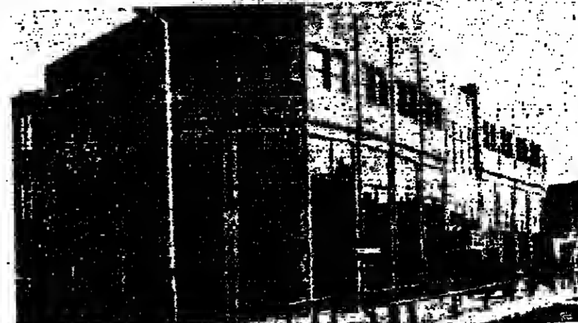
Canada Life has completed its second direct British office development in Kingston upon Thames. Located in the heart of the town's conservation area, Berkeley House provides 15,600 sq ft of air conditioned offices on ground, and three upper floors together with parking for 30 cars. Joint letting agents Clive Lewis & Partners and Weatherall Green & Smith are asking £11.54 a sq ft rent.
